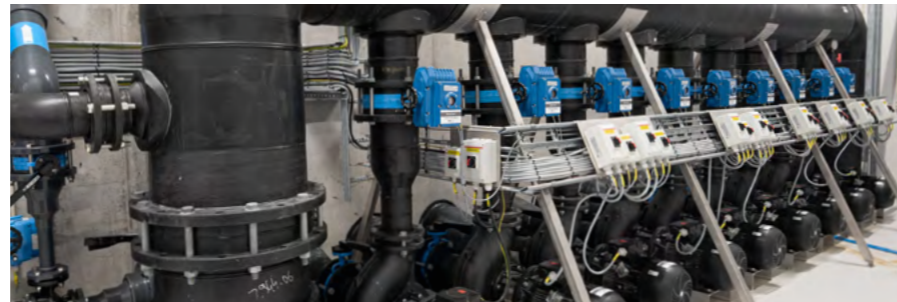
Figure 27 - Main pump manifold with 9 pumps for circulation of RAS water
